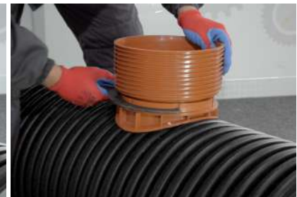
12. Final tightening of sag
