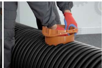
8. setting the spacer ring
