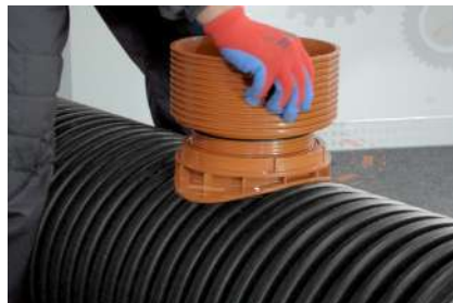
11. Setting the selected connection
