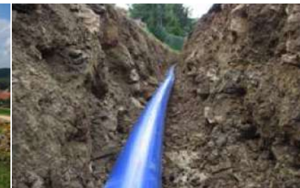
Installation without sand bedding
