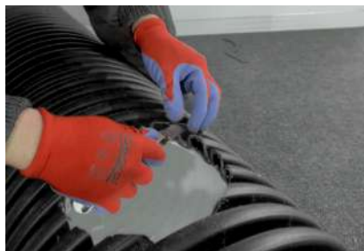
5. Cleaning chips and forming a clear hole
